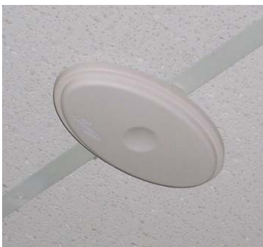
Installed Antenna
